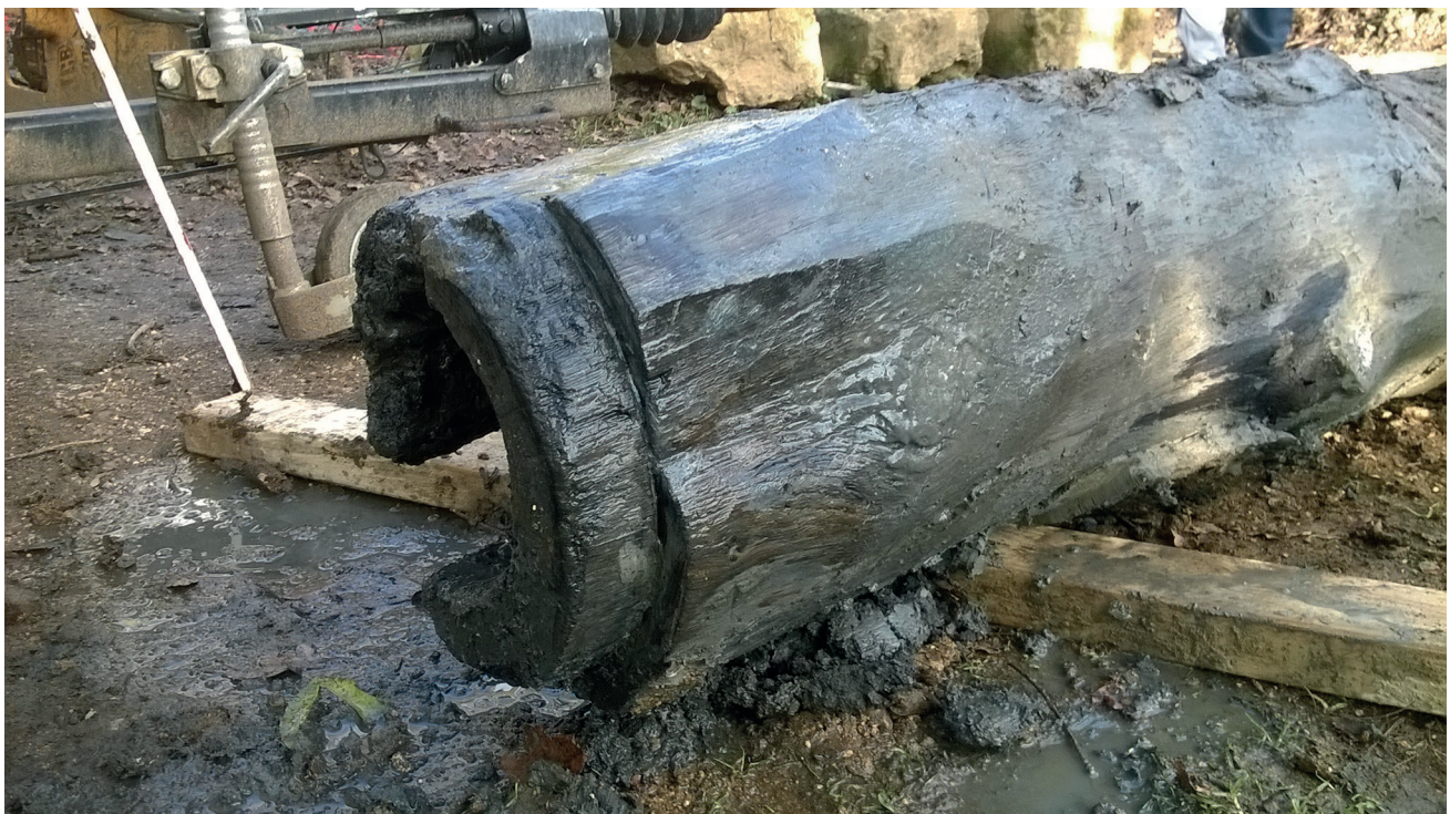
Figure 10: The substantial Oak water pipe
