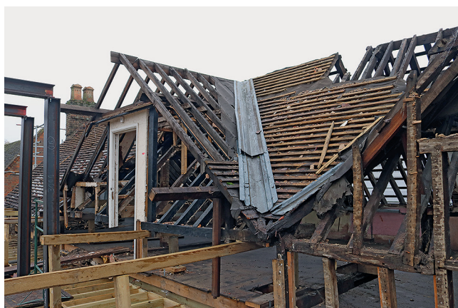
Figure 11: View of the roof during works to 18–20 St Peter's Street, Bedford.
