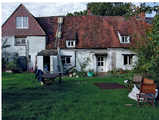
Figure 4: Rear of house and location of test pit DC17
