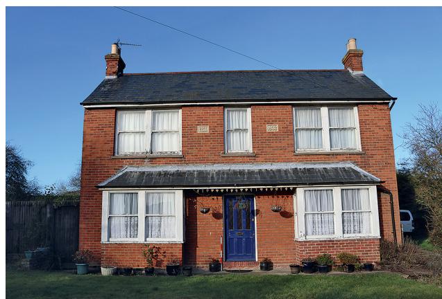
Figure 12: No. 100 High Street, Meppershall.
