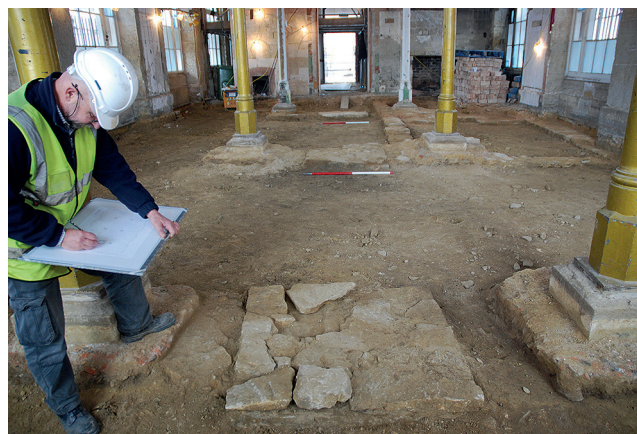
Figure 6: Brackley Town Hall during excavations
